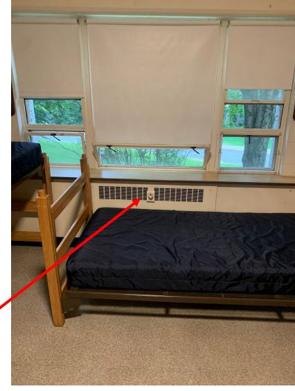
Locate your thermostat controller. In many dorm rooms, it is mounted directly on the heater cabinet face or on the piping attached to the heater. It could be hidden behind the bed or furniture. Please become familiar with its location as you may need to adjust during cold weather.
