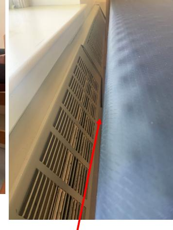
The bed appears to be touching the heater, and a bedspread can be covering up the open slats on the heater face. Pulling the bed away from the heater a few inches to keep the slats free for air movement is advised.
