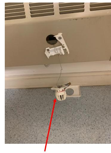
Destroyed controller most likely from furniture being moved. This can lead to room overheating or room underheating.
